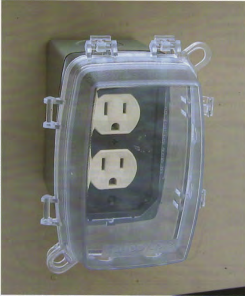
Photo 2. This cover is weatherproof even with a cord-and-plug connection in use.
