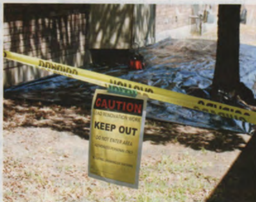
For this bay-window repair, the author covered the ground with 6-mil plastic (above), using stakes and plastic clips to keep the sheet secure (above right), then set up warning tape and posted signs (right).
