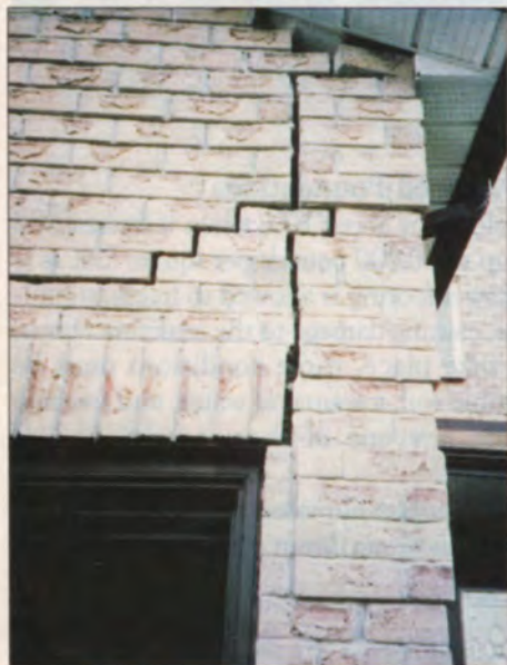
Figure 2. Unheated garages are prone to damage from adfreezing (left). Two layers of 6-mil polyethylene placed on both sides of the foundation wall provides a slip plane that prevents freezing soils from bonding to the foundation wall (right).
