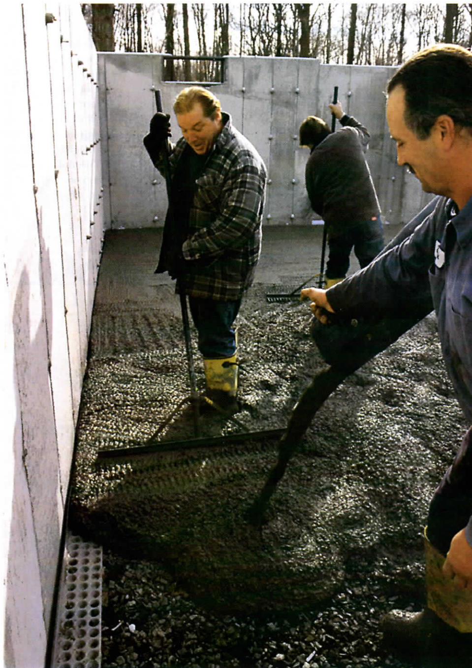
Drainage flashing is a simpler, less expensive interior drain. Installed at the junction of wall and footing, this flashing has a dimpled profile that allows any water from the walls to flow beneath the slab and into the sump pump. Obviously, it's important to keep the top of the flashing clear when pouring the slab (photo right).
