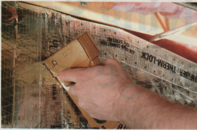
Figure 6. The female end of a duct board joint is pulled taut and stapled through to the male end (left). The joint is completed by applying heat-activated tape, which is warmed with an Amcraft duct board iron (right).
