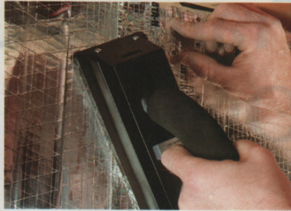
Figure 6. The female end of a duct board joint is pulled taut and stapled through to the male end (left). The joint is completed by applying heat-activated tape, which is warmed with an Amcraft duct board iron (right).
