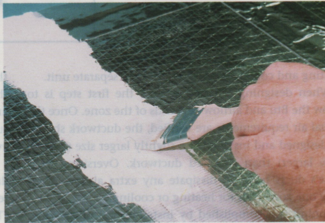
Figure 5. Joints in sheet-metal duct should be sealed with mastic, which can be applied with a paint brush (left). When mastic is used on duct board, the joint should first be bridged with fiberglass tape or scrim (right).
