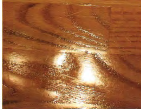
Sloppy sanding shows. Using a worn sanding screen to sand between coats of finish can leave spiderweb-like defects in floor finish.
