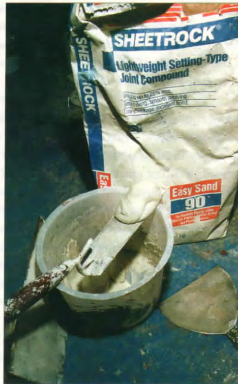
Plaster crack repair is a valuable skill for any old-house owner, and the tools are minimal and simple. Left: A sponge is useful for clean-up. Right: Beginners will find a setting-type compound easier to apply than plaster. The authors use a 6" joint-compound knife for the important infill step.
