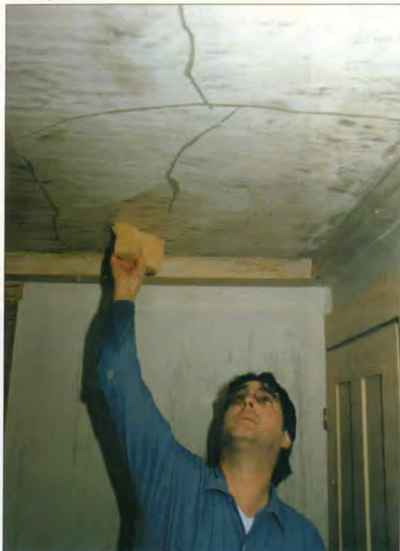
Plaster crack repair is a valuable skill for any old-house owner, and the tools are minimal and simple. Left: A sponge is useful for clean-up. Right: Beginners will find a setting-type compound easier to apply than plaster. The authors use a 6" joint-compound knife for the important infill step.
