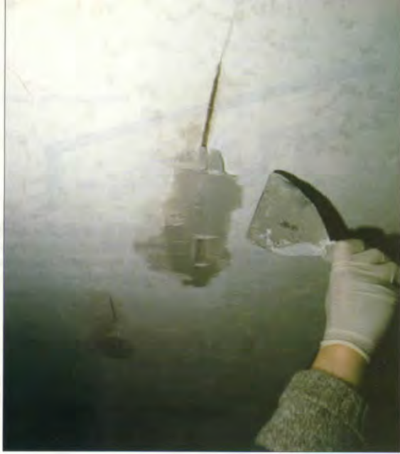
Above: Applying the first coat of compound from both sides to push it well into and under the crack. Right: Applying the second and third coats, the knife is held almost on end to scrape off excess.
