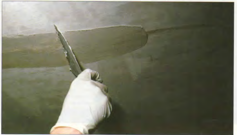
Above: Applying the first coat of compound from both sides to push it well into and under the crack. Right: Applying the second and third coats, the knife is held almost on end to scrape off excess.
