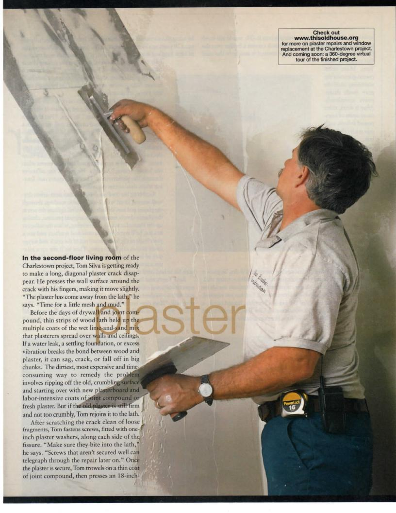
wide strip of fiberglass insect screening into it. (He would use mesh joint tape for a smaller area.) "The mesh creates a bridge over the crack, to bond to the stable plaster around it and hold the mud
