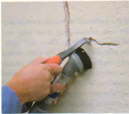
Cyclical cracks are the bane of antique plaster walls and must be repaired with care to avoid reoccurrence. First, dig out the crack in an inverted V (left) that undercuts the plaster, vacuuming out all debris. Next, thoroughly wet the crack with water, then apply bonding agent with a brush at the undercut edges to help new plaster bond to the old. Then fill with patching plaster to slightly proud of the surface and sand flush when dry.
