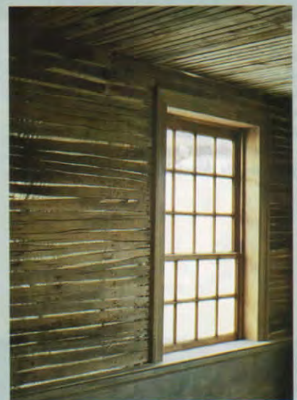
ABOVE: Pre-industrial plaster is marked by irregular lath, such as "accordion" lath, hand split from thin boards. BELOW: With industrialization, lath became more regular, from early saw lath (right in photo) to fully mass-produced lath and nails.
