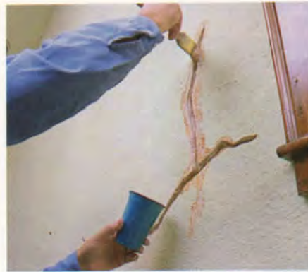
Cyclical cracks are the bane of antique plaster walls and must be repaired with care to avoid reoccurrence. First, dig out the crack in an inverted V (left) that undercuts the plaster, vacuuming out all debris. Next, thoroughly wet the crack with water, then apply bonding agent with a brush at the undercut edges to help new plaster bond to the old. Then fill with patching plaster to slightly proud of the surface and sand flush when dry.
