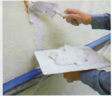
Cyclical cracks are the bane of antique plaster walls and must be repaired with care to avoid reoccurrence. First, dig out the crack in an inverted V (left) that undercuts the plaster, vacuuming out all debris. Next, thoroughly wet the crack with water, then apply bonding agent with a brush at the undercut edges to help new plaster bond to the old. Then fill with patching plaster to slightly proud of the surface and sand flush when dry.
