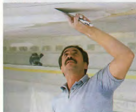
For finish coats, patching compound is okay for small areas, but finish plaster is preferred for large holes. Do your best to match the overall character, as a patch that's too rough—or too smooth—may be obvious under paint.
