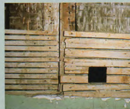
ABOVE: Pre-industrial plaster is marked by irregular lath, such as "accordion" lath, hand split from thin boards. BELOW: With industrialization, lath became more regular, from early saw lath (right in photo) to fully mass-produced lath and nails.
