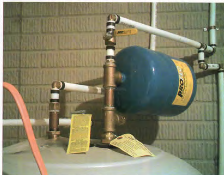
Control thermal expansion. An expansion tank, such as the one shown above, helps to absorb water pressure that results from thermal expansion. The tank can be installed anywhere in the cold-water line between the house's main valve and water heater, or on the hot-water line within 3 ft. to 5 ft. of the water heater. An expansion tank should be installed in conjunction with a pressure-reducing valve in high-pressure situations.
