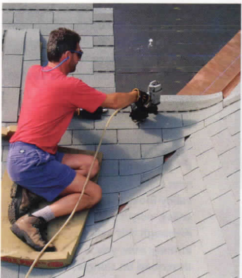
Nail now, cut later. A second way to install the shingles in an open valley is to run them long through the valley (photo left). Then, after snapping a cutline, trim the shingles with a hook blade in a utility knife, using sheet metal to protect the valley liner (photo right).
