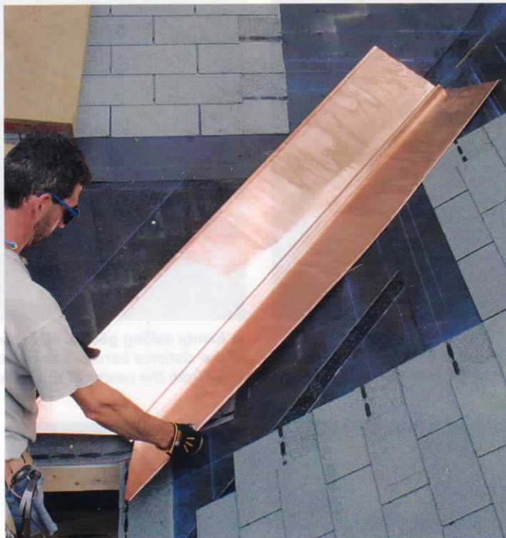
An extra crimp for extra protection. An inverted V in the center of the valley liner helps to channel water down the valley while allowing for expansion and contraction widthwise.
