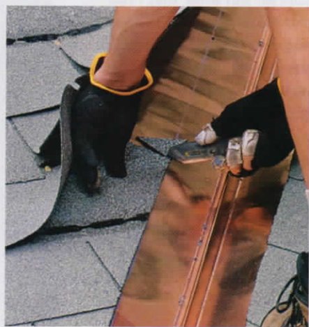
Dubbing corners can prevent leaks. Dubbing or clipping the corners of shingles along the valley keeps water flowing downhill along a cut edge. Corners can be clipped either before the shingles are installed or in place before the edge is cemented.
