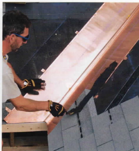
Start spreadin' the goo. If you cut the shingles before nailing them in, spread a band of roof cement on the metal liner first (photo left). As each course goes on, the roof cement is spread on the top lap of each shingle as well (photo right).
