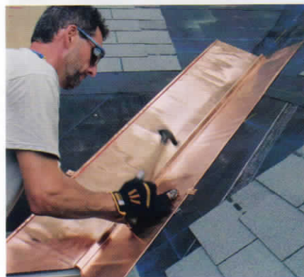
Two ways of holding down the liner. To allow the liner to expand lengthwise, fasteners cannot be driven through the liner. Instead, nails can be driven snug along the edge of the liner (photo right), or simple clips can engage a hem along the edge (photo left).
