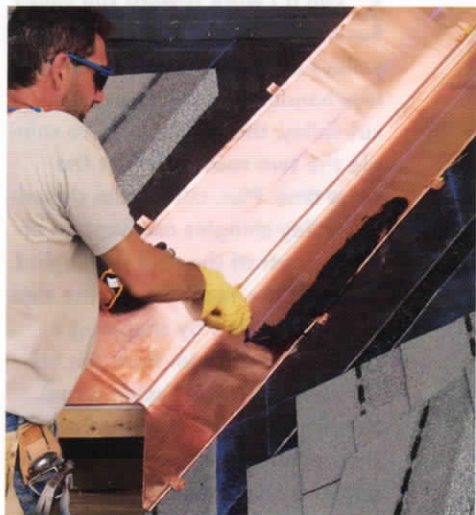
Start spreadin' the goo. If you cut the shingles before nailing them in, spread a band of roof cement on the metal liner first (photo left). As each course goes on, the roof cement is spread on the top lap of each shingle as well (photo right).
