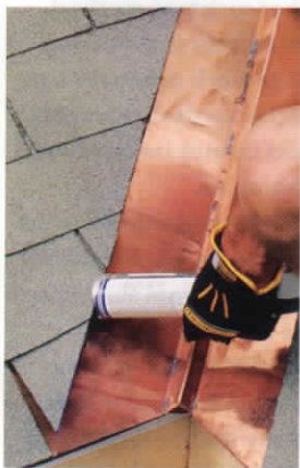
A controlled double bead. For a quick and easy double bead of sealer, run the first bead with the nozzle of the gun inserted all the way under the shingles (photo left). A finger on the nozzle spaces the second bead (photo center), and the beads continue on the top lap of each shingle to complete the seal (photo right).
