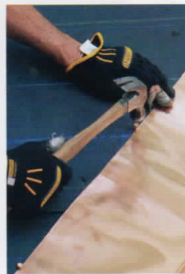
Two ways of holding down the liner. To allow the liner to expand lengthwise, fasteners cannot be driven through the liner. Instead, nails can be driven snug along the edge of the liner (photo right), or simple clips can engage a hem along the edge (photo left).
