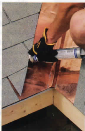
A controlled double bead. For a quick and easy double bead of sealer, run the first bead with the nozzle of the gun inserted all the way under the shingles (photo left). A finger on the nozzle spaces the second bead (photo center), and the beads continue on the top lap of each shingle to complete the seal (photo right).
