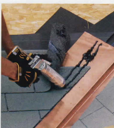
A controlled double bead. For a quick and easy double bead of sealer, run the first bead with the nozzle of the gun inserted all the way under the shingles (photo left). A finger on the nozzle spaces the second bead (photo center), and the beads continue on the top lap of each shingle to complete the seal (photo right).
