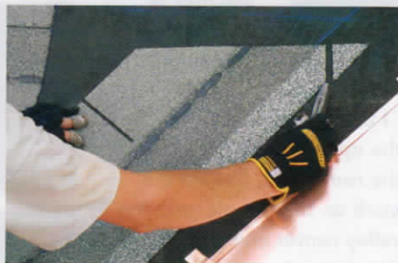
Dubbing corners can prevent leaks. Dubbing or clipping the corners of shingles along the valley keeps water flowing downhill along a cut edge. Corners can be clipped either before the shingles are installed or in place before the edge is cemented.
