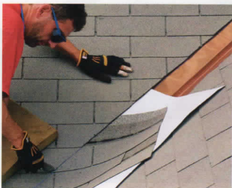
Nail now, cut later. A second way to install the shingles in an open valley is to run them long through the valley (photo left). Then, after snapping a cutline, trim the shingles with a hook blade in a utility knife, using sheet metal to protect the valley liner (photo right).
