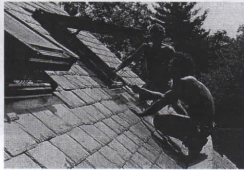
Pretenders on the slate scene are mineral fiber roofing shingles from Supradur Manufacturing Corp. Shunned by authentic slaters, Supra-Slate fiber reinforced concrete shingles are nevertheless making inroads as a substitute for the real thing. Approaching its 75th anniversary, The Wagner Roofing Company seeks out workers who have some interest in learning the trade and then trains them on the job.
