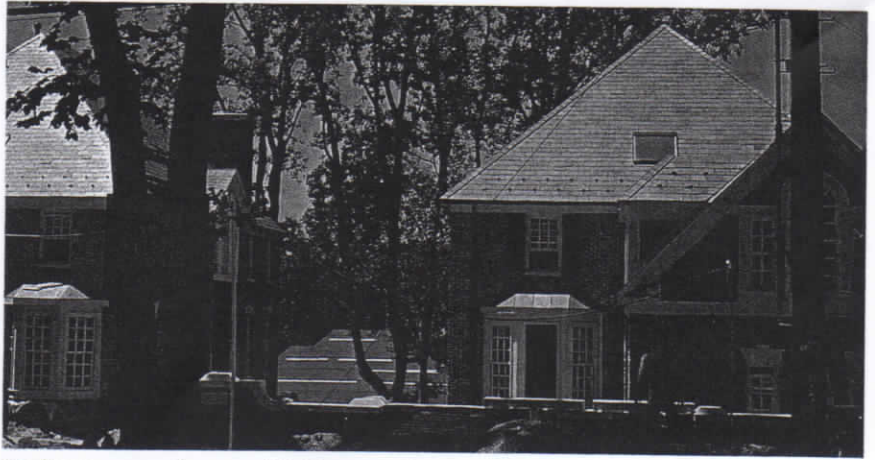
Roofing two new homes with Vermont slate.
