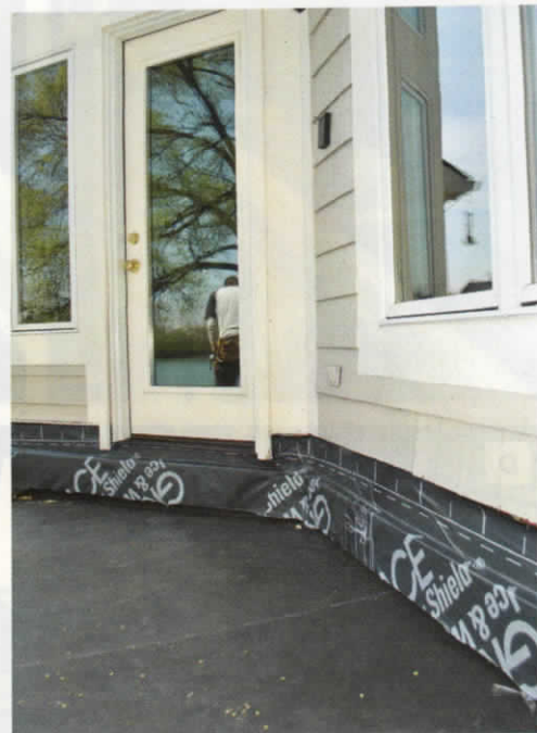
Figure 7. A pressure-treated deck ledger (above left), flashed with Ice & Water Shield (above), supports the inboard end of the new joists. The original decking and railing were reinstalled to complete the roofing job (left).
