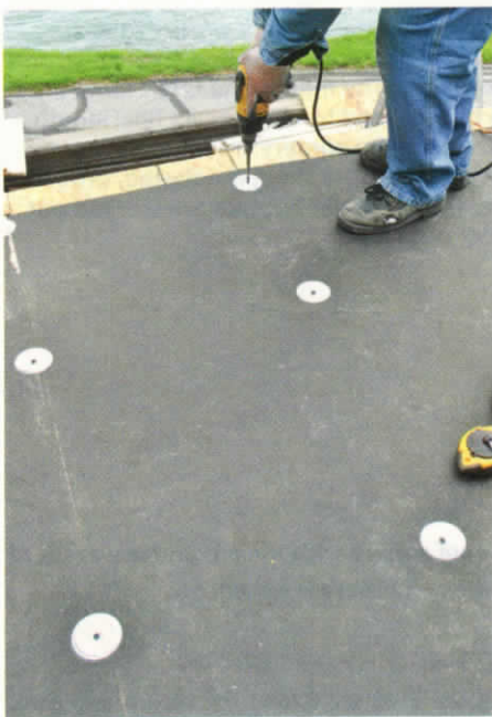
Figure 3. The EPDM installation started with a 1/2-inch-thick fiberboard underlayment engineered to bond with the roofing adhesive. It scores and cuts like cement board and is fastened in place with galvanized screws and washers (above). After sweeping the surface clean, the crew applies latex bonding adhesive, folding the membrane back on itself so it can be glued down a section at a time (right).
