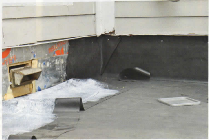
Figure 4. As the cement sets, a worker uses a broom to press out air bubbles and create a strong bond (above left). The membrane is left long, then folded up the wall and trimmed to its final length. To minimize cuts, the corners are folded over (above). After the entire sheet is adhered, brooming continues until all the bubbles are worked out at the upper edge (left).
