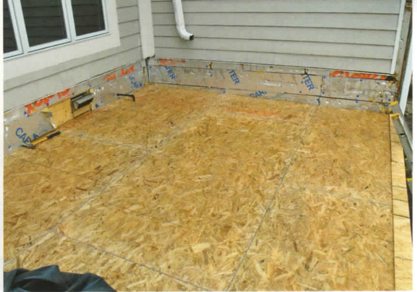
Figure 2. Since the sheathing had to be replaced anyway, the author increased the roof slope by adding tapered 2-by sleepers on top of the joists (left). The new OSB decking slopes 4 inches over 11 feet — an additional 3 inches of rise (above).
