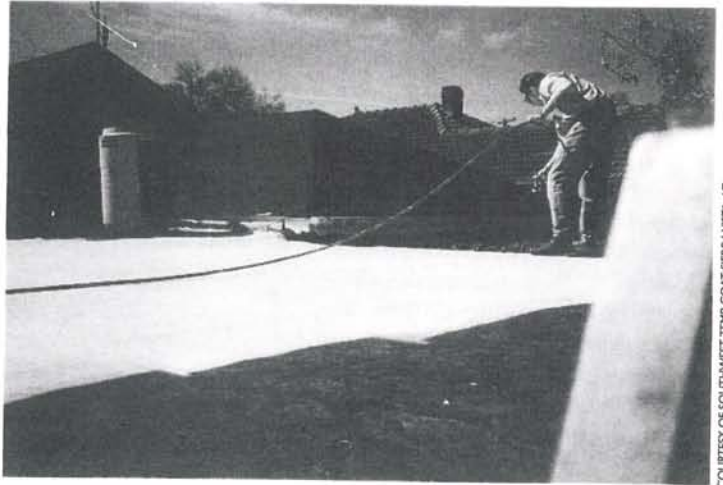
White roof coatings with high solar reflectance can be applied over asphalt shingles and most other roofing materials.
