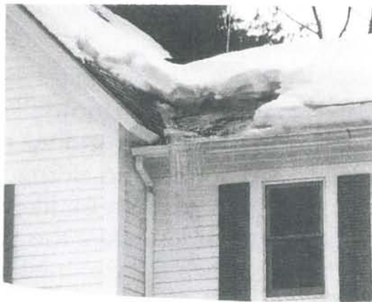
Homeowners should plan ahead for the winter months when embarking on a reroofing project. The ice dams on the edges of these roofs, and the bare spot created by leaking heat in the photo on the left, show that additional weatherization is needed. Through adequate insulation, air sealing, and attic ventilation, existing homes can be effectively retrofitted.
