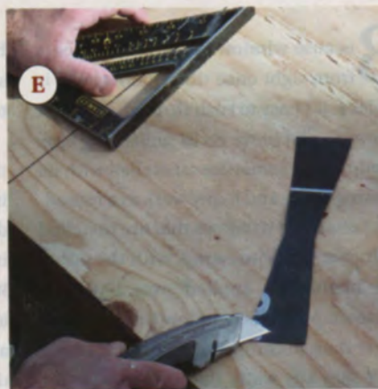
Figure 2. Transferring the dimensions of the flashing pieces to a plywood story board makes it easier to cut them accurately to length (A). Each piece is then folded lengthwise twice (B) so it's short enough to cut against a standard framing square (C). Corner pieces, or bow ties — measuring about 1½ inches by 8 inches overall — are cut from scrap material (D, E).
