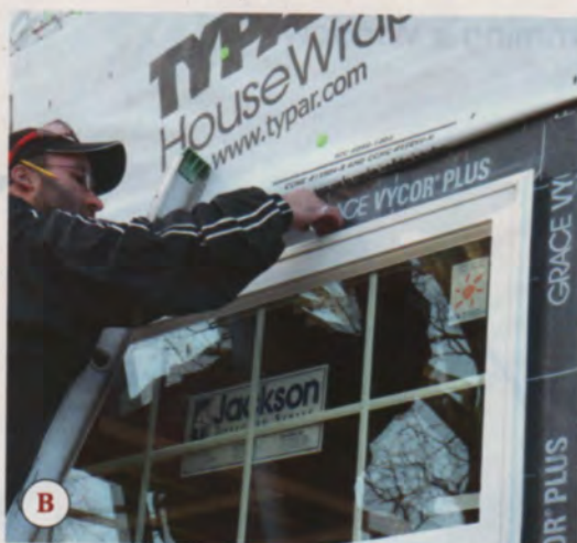
Figure 7. Outer flashing goes on over the window's side and top flanges (A, B). The flap of housewrap above the window head is then pulled down and taped in place over the head flashing (C, D).
