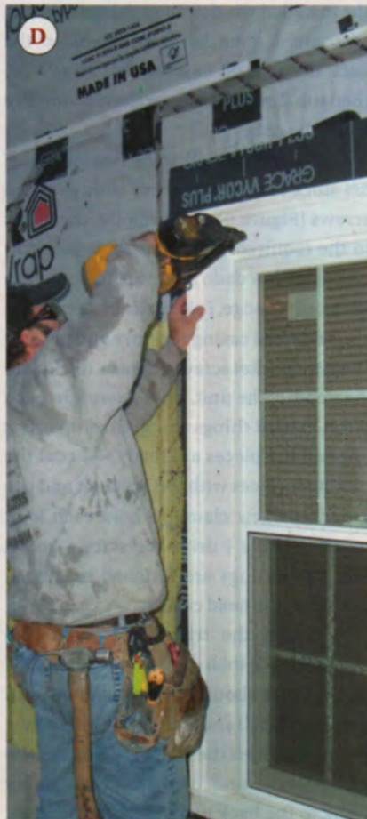
Figure 11. Once the trim unit has been tacked in place and leveled, the screws are driven home, starting at the bottom (A, B). A PVC trim band covers the outer row of screws (C, D); the remaining holes are plugged.
