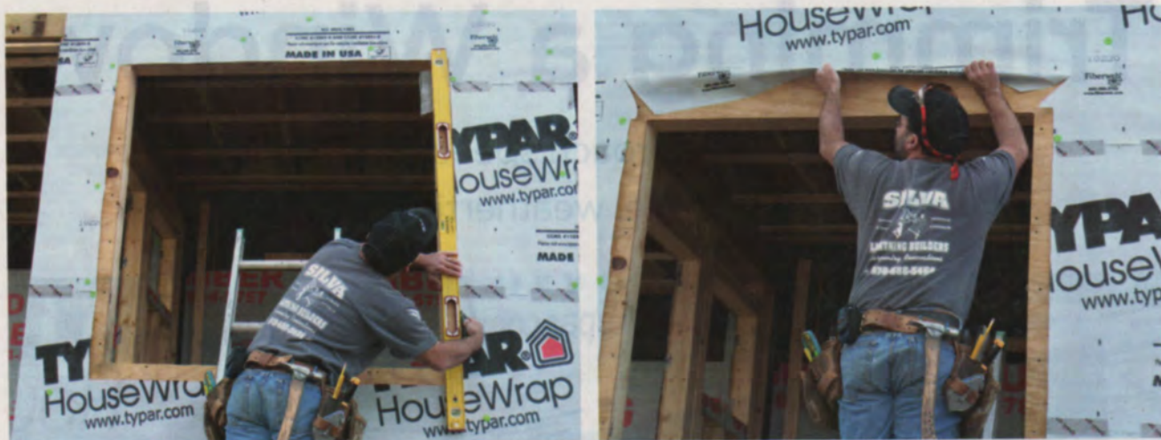
Figure 1. Once the housewrap has been cut back from the sides and bottom of the rough opening by the width of a level (left), a flap along its upper edge is temporarily tucked out of the way (right).
