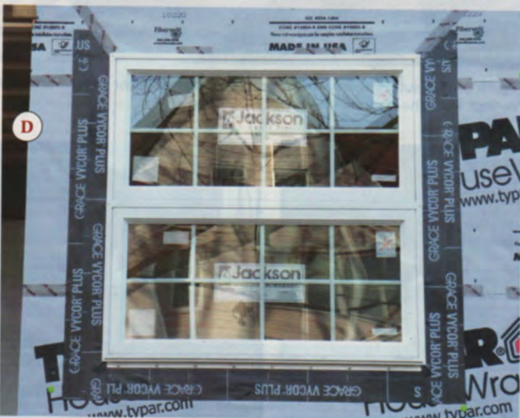
Figure 7. Outer flashing goes on over the window's side and top flanges (A, B). The flap of housewrap above the window head is then pulled down and taped in place over the head flashing (C, D).
