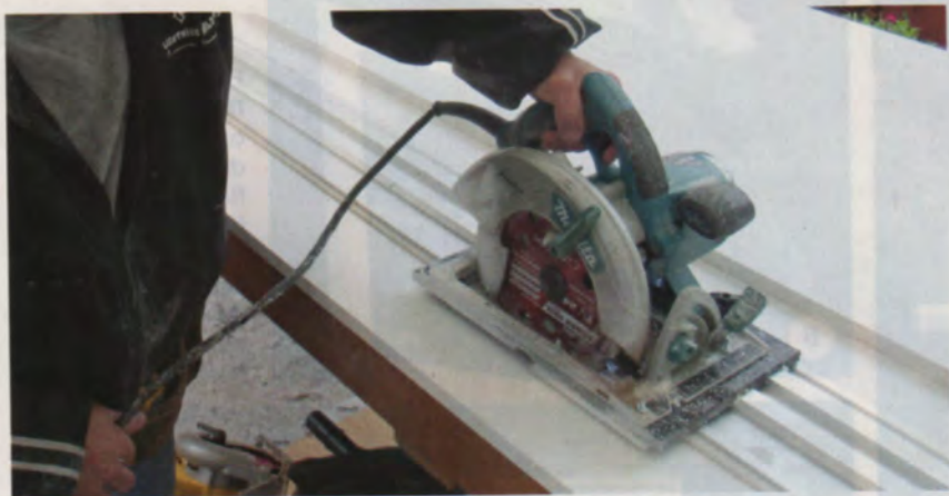
Figure 8. The author uses a track saw to create exterior trim of any width from 3/4-inch PVC sheet stock.
