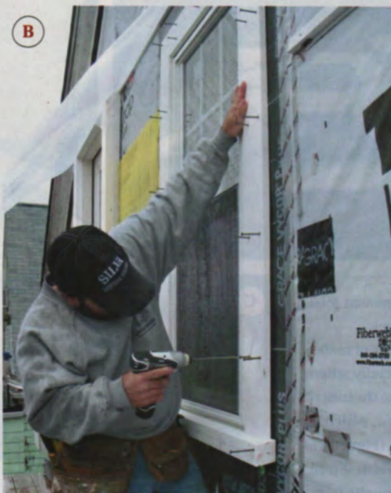
Figure 11. Once the trim unit has been tacked in place and leveled, the screws are driven home, starting at the bottom (A, B). A PVC trim band covers the outer row of screws (C, D); the remaining holes are plugged.
