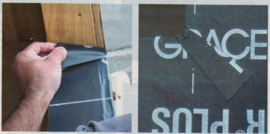
Figure 4. One end of a bow tie is adhered to the flashing membrane outside the opening, the other half folded to the inside (left). When applied correctly, the narrow center section will turn neatly up the corner of the opening (right).
